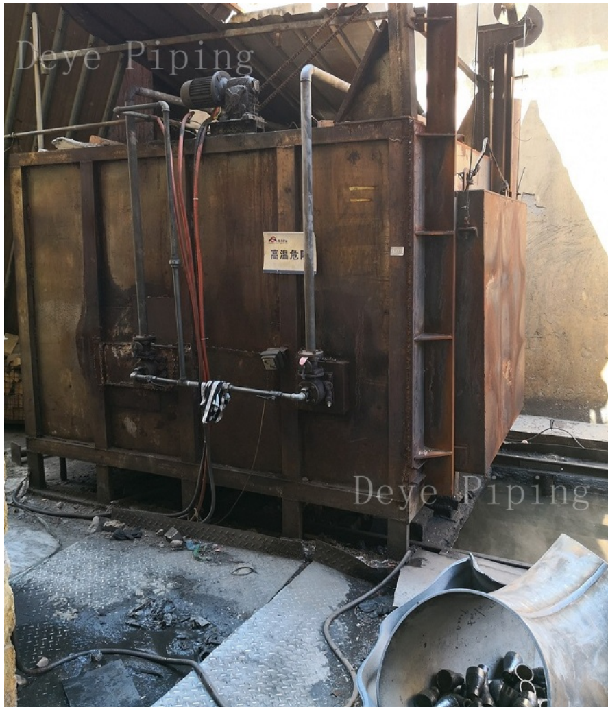
6. Shot Blast and cleaning
